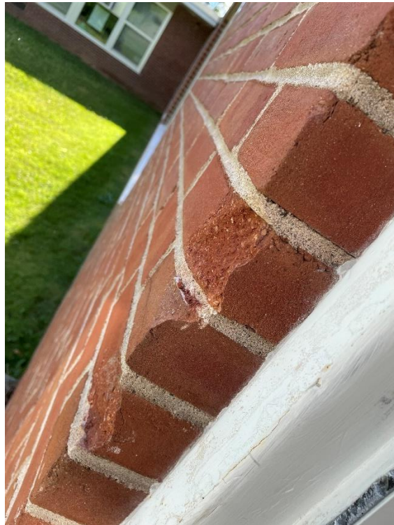
Exterior Brick & Mortar
