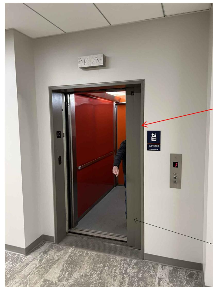
SCRAPE AND CLEAN EXISTING ELEVATOR HOISTWAY DOOR FRAMES AND PROVIDE NEW ELECTROSTATIC PAINT FINISH TO MATCH EXISTING COLOR, TYP FOR BUILDING
