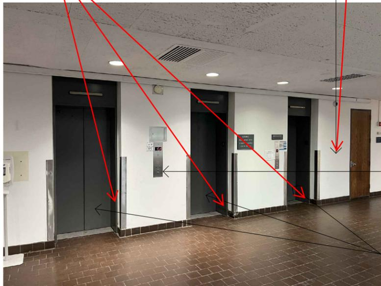
SCRAPE AND CLEAN EXISTING ELEVATOR HOISTWAY DOOR FRAMES AND PROVIDE NEW ELECTROSTATIC PAINT FINISH TO MATCH EXISTING COLOR, TYP FOR BUILDING
