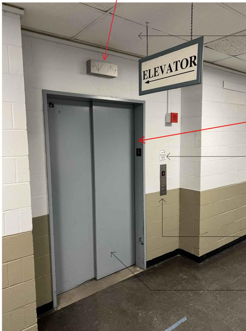
REMOVE ACT CEILING TILE AS NEEDED TO COMPLETE THE WORK AND STORE TO BE REINSTALLED. REINSTALL ACT CEILING TILES AFTER NEW CONDUIT AND PIPING INSTALLATION.
