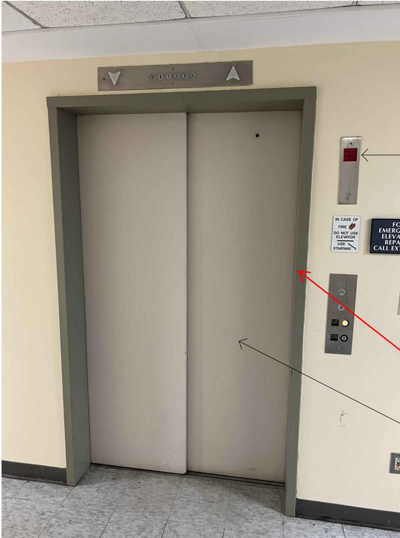
REFER TO ELEVATOR DRAWINGS & SPECS FOR INFORMATION ON DEVICE UPGRADE/REPLACEMENT, PATCH/REPAIR ADJACENT WALL SURFACES AS PART OF NEW DEVICE INSTALLATION (TYP)
