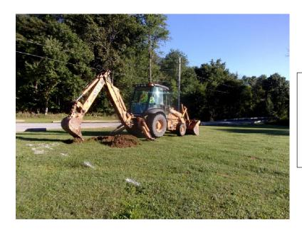
PHOTO 2: View of the northeast building corner, starting to excavate Test Pit 2. The entrance road crosses a small tributary to Moodna Creek about 200 feet east from end of the proposed building.
