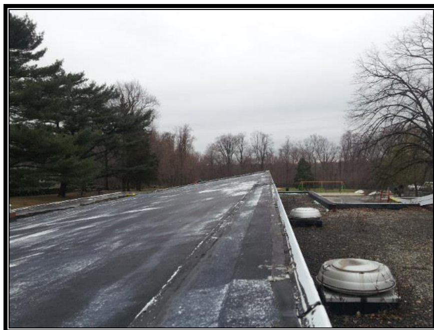
Photograph 1: Roof Area - Roofing Material.
