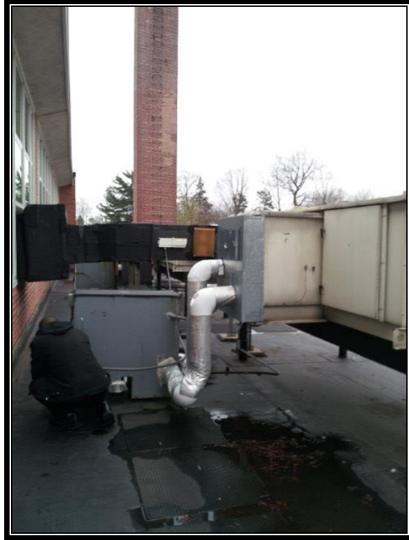
Photograph 3: Roof Area – Paper to Ductwork Fiberglass Insulation & AC Unit Caulking.
