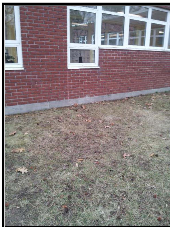
Photograph 2: Exterior Façade – Exterior Expansion Wall Joint & Exterior Brick Mortar.
