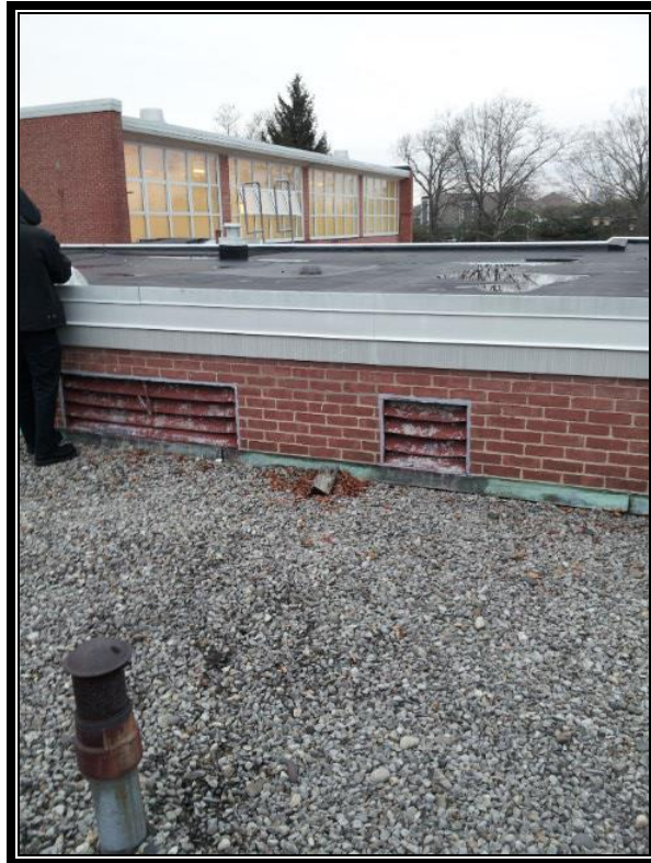
Photograph 4: Roof Area - Louver Caulking.
