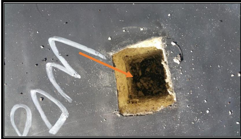
**Photograph 1: Typical Roofing System for Roofs A, B & C – Tar on Concrete, Roofing Felt Paper, Roofing Rubber Membrane w/ Glue & Tar on Roofing Membrane.**
