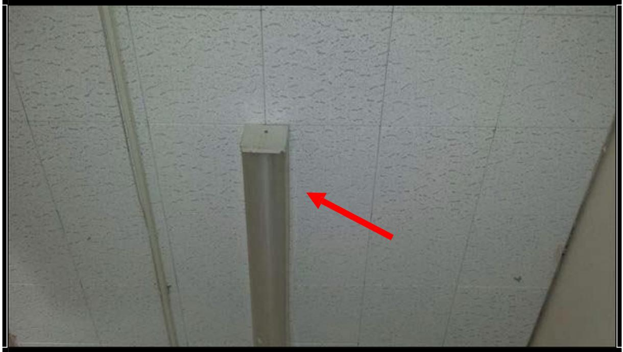
Photo # 03: 1'x1' Gouged Ceiling Tile, White
