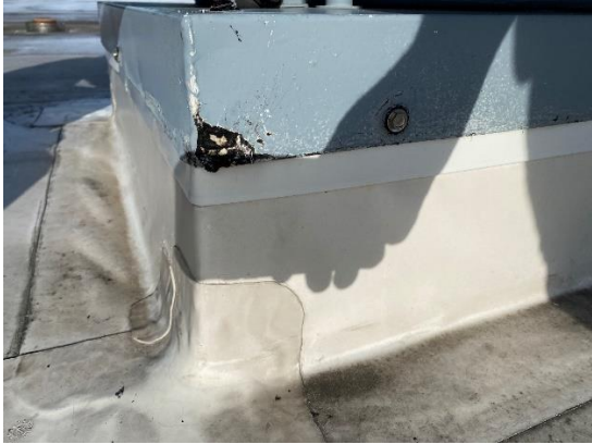
HVAC Vent Caulk – Black
