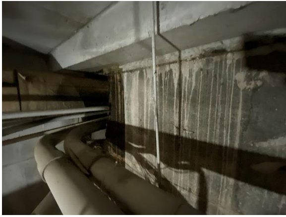
Crawl Space Below 1 st Floor
