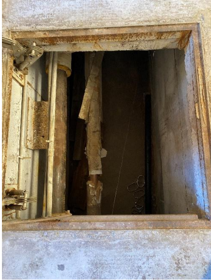
Man Hole to Crawl Space
