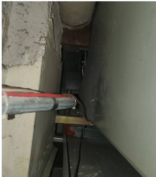
Photo #2 – Available Space for Maintenance Access
