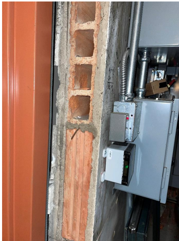
Partition Build Up
