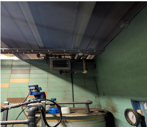
Photograph 3 – 016-01 White Mudded Fittings
