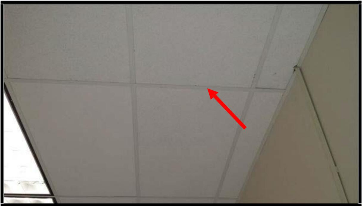
Photo # 04: 2'x4' Small Pinhole Ceiling Tile, White
