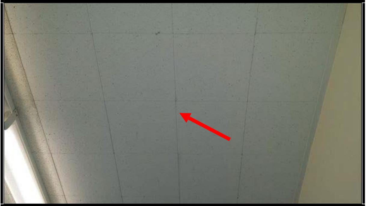
Photo # 05: 1'x1' Fissured Ceiling Tile, White
