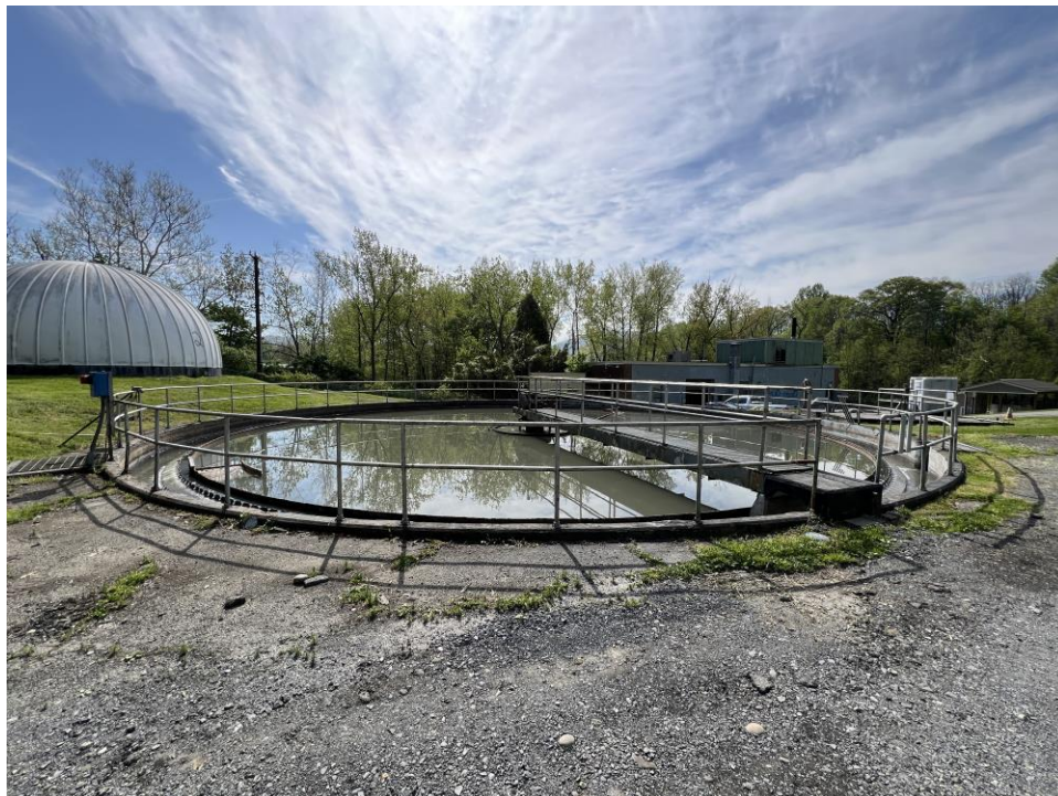
Photo – Example of LBP Outer Railing (Primary Tank 1, 2, & Trickling Filter 2) – Metal Railing – Gray LBP
