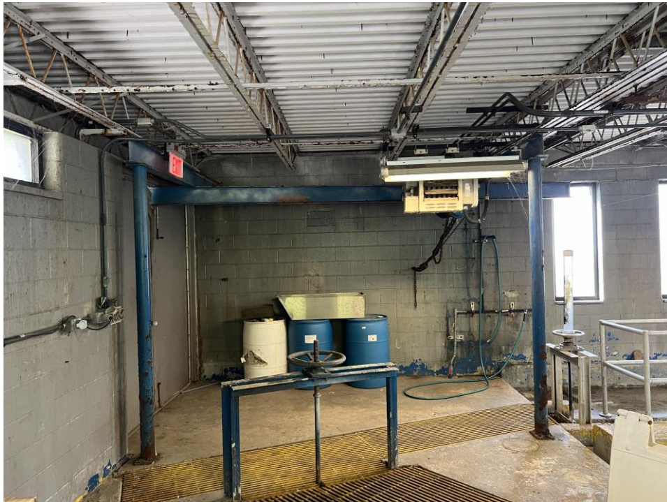
Photo – Example of LBP Outer Railing (Primary Tank 1, 2, & Trickling Filter 2) – Metal Railing – Gray LBP
