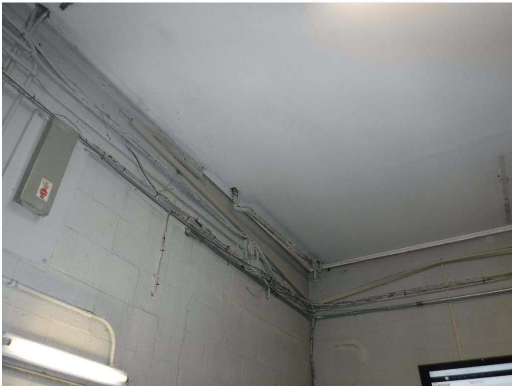
Original Building: Asbestos containing ceiling gypsum board and joint compound.
