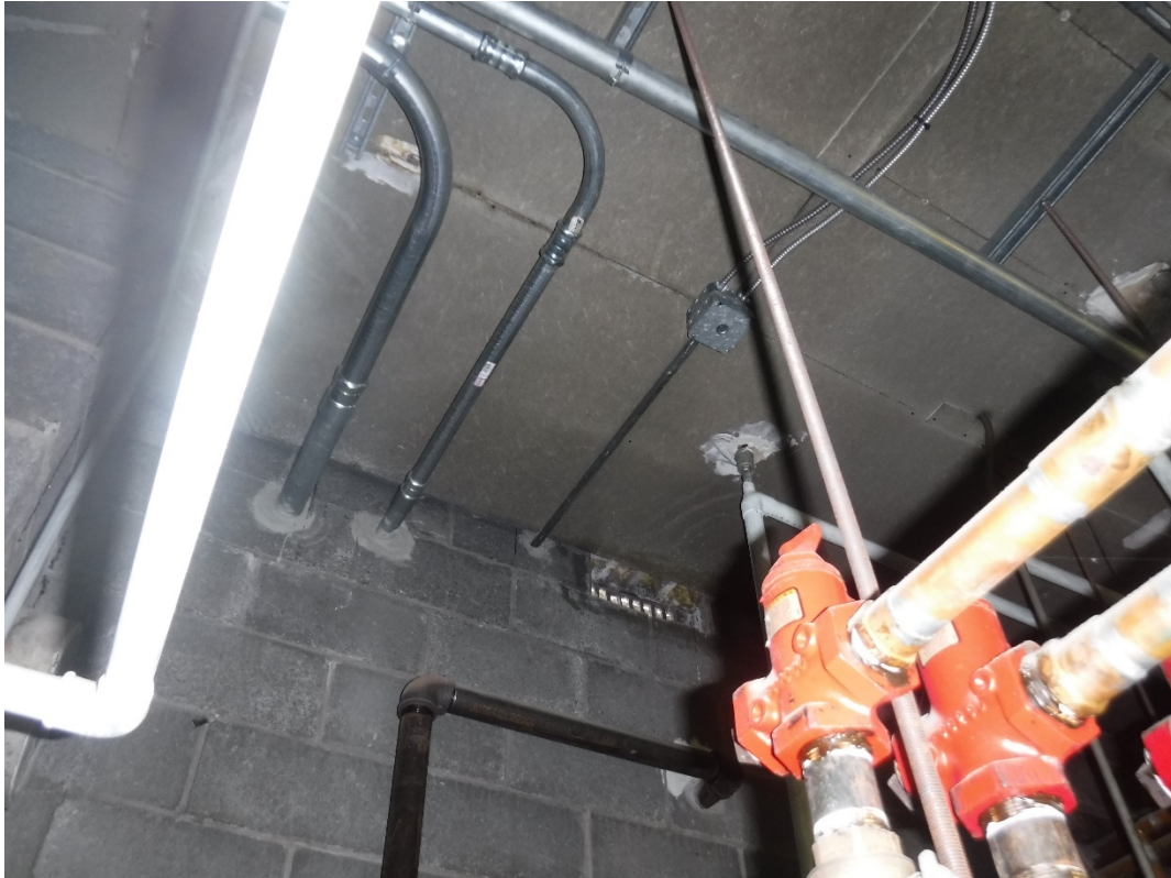
Boiler Room: Asbestos containing transite ceiling.
