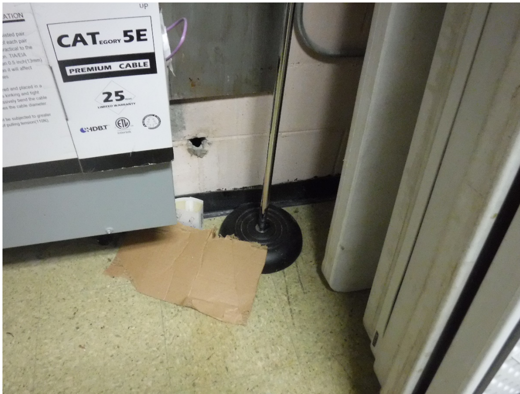
Bar Storage: Asbestos containing black cove base and mastic.
