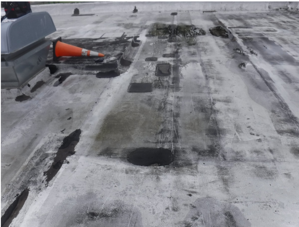
New Building Exterior Roof: Asbestos containing HVAC flashing, and parapet flashing. Non-asbestos containing seam tar, top of parapet tar.
