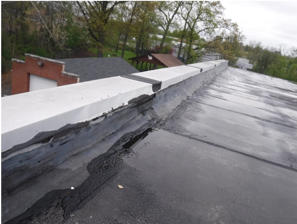
New Bay Roof: Asbestos containing parapet flashing.
