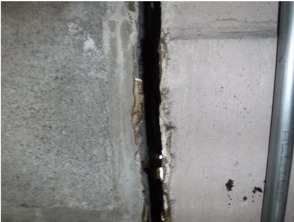
Attached shed: Asbestos containing gap caulk.
