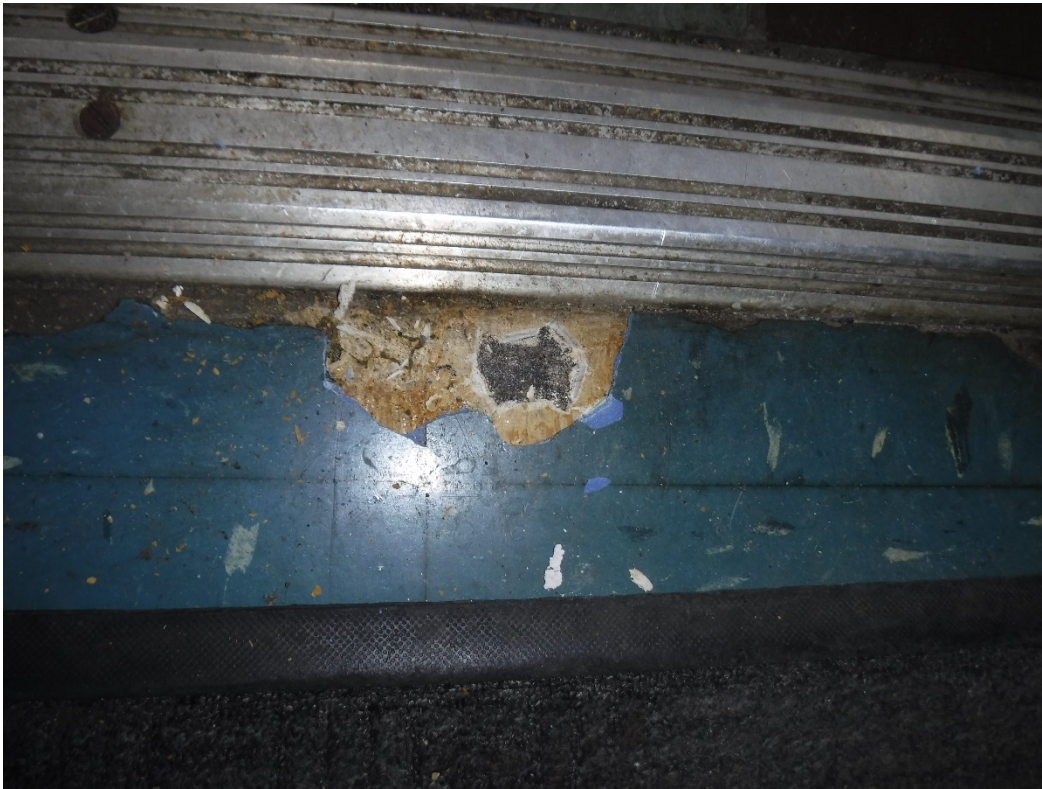
Meeting Room: Asbestos containing vinyl floor tile (bottom layer) and associated mastic.
