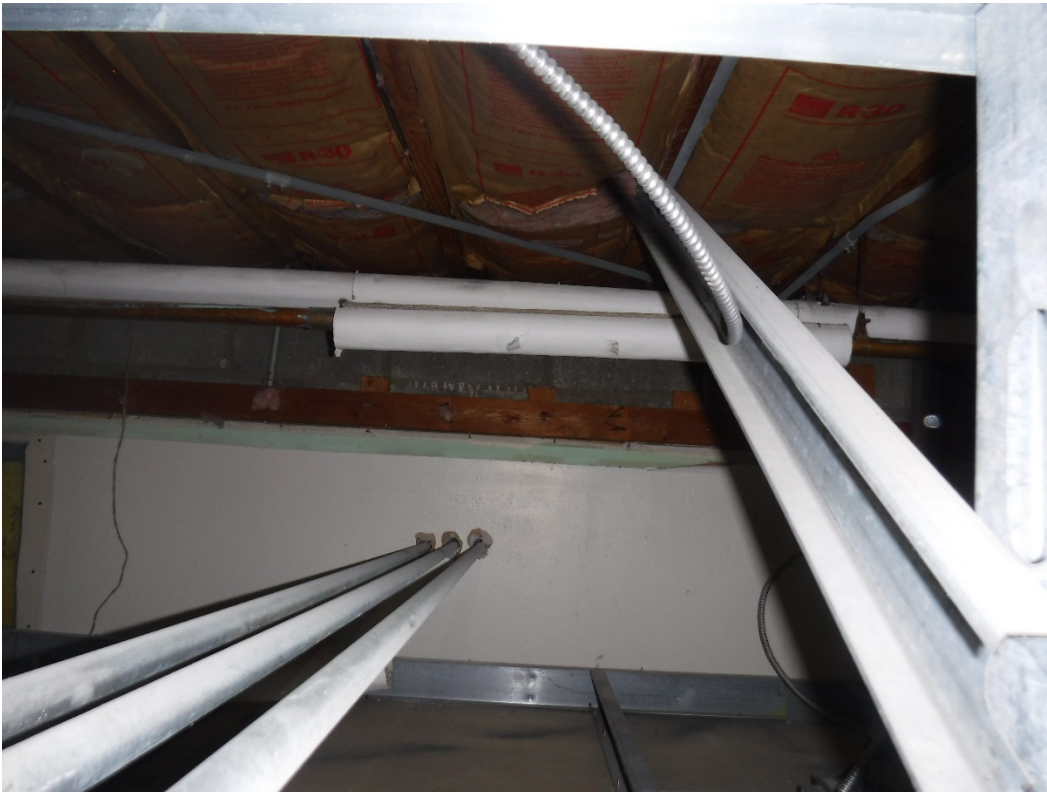
Meeting Room: Asbestos containing pipe insulation (above soffit ceiling).
