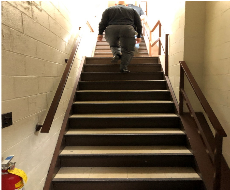
2 nd Floor: Asbestos containing 12"x12" tan vinyl floor tile.
