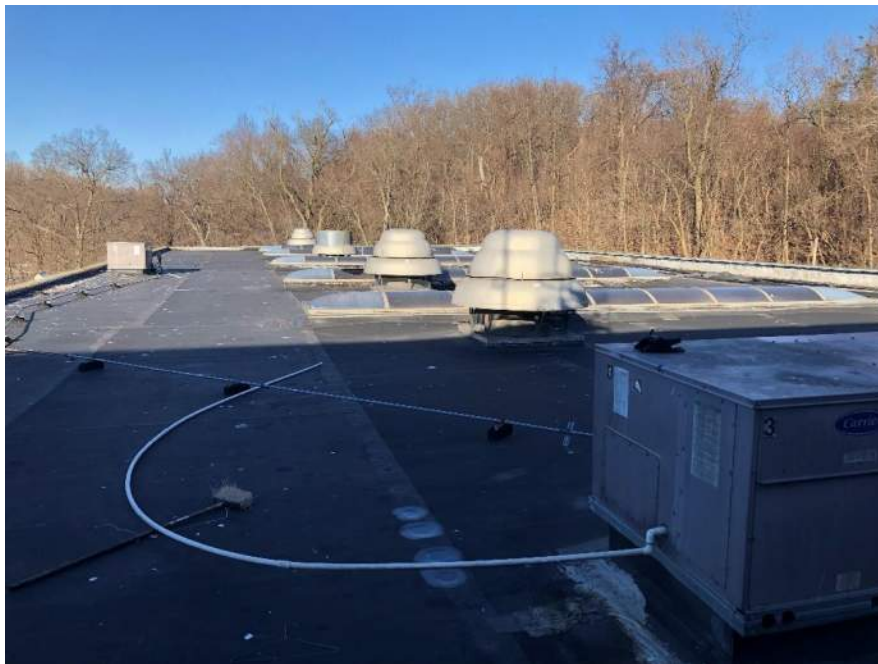
Photo 1 – Overall view of Transfer Station roof.
